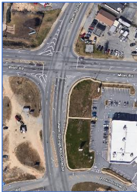
Miller Rd Intersection
